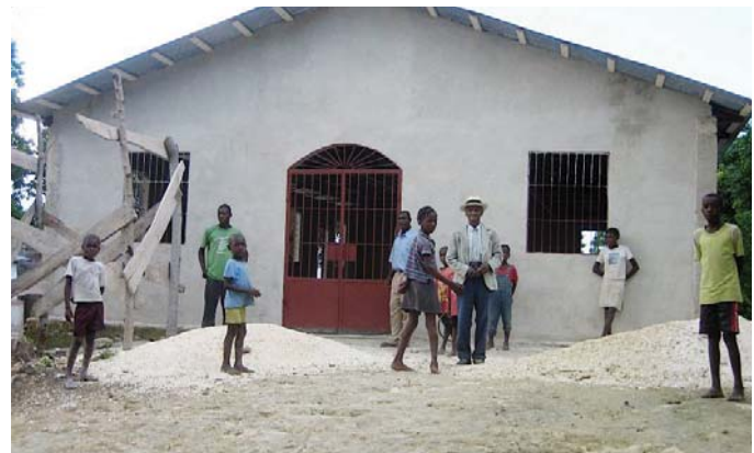
New Boyer church. Thanks for giving, and the work teams who worked so hard to make this project possible.
